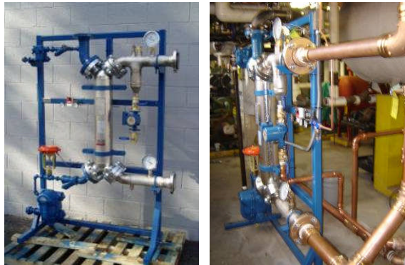
Duplex 60 gpm Domestic Water on 60 psi steam
